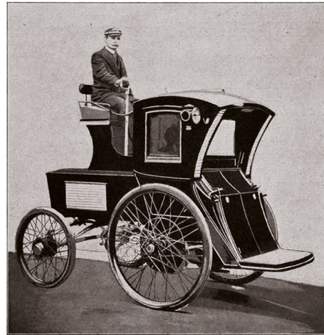
FIGURE 2 Electric trolley of the Electric Carriage & Wagon Company (© Springer Vieweg)
